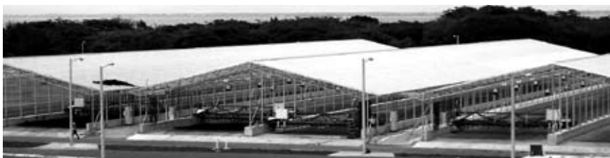
Figure 1: Panoramic view of the entire solar sludge drying plant
