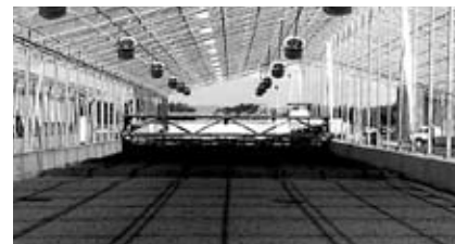
Figure 2: WendeWolf® machine completely installed in a greenhouse
